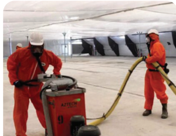
On-tool dust extraction for floor grinding
