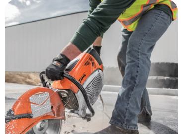
Water suppression for cutting
